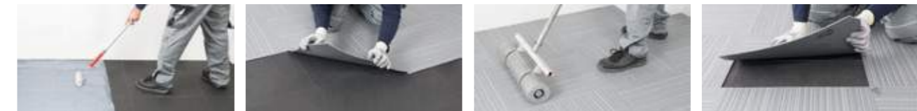
Installation with tackifier
