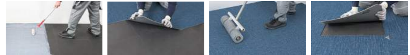
Installation with tackifier
